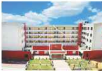
Apex Central Campus Near Assembly, Nakul Path, Lal Kothi Scheme, Tonk Road, Jaipur
