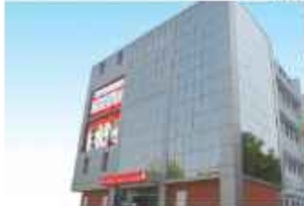
Apex West Campus - II Shilpa Path, Near Technology Park, Mansarovar, Jaipur-302020
